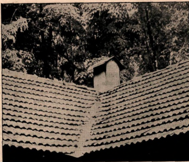
The roofing of the smoke house with the Chimney. (The smoke house is built in the corner of two wings constituting store, coagulating and machining shed and office).
