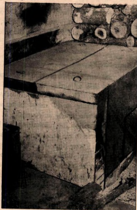
The outer top casing without cracking even after use for over 12 years.
