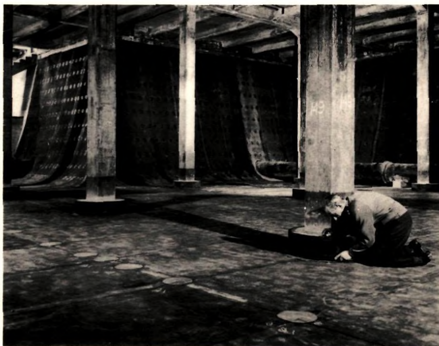
Part of the 25 - million - gallon reservoir at Easington, with a General Rubber Goods Division expert at work on the lining.
