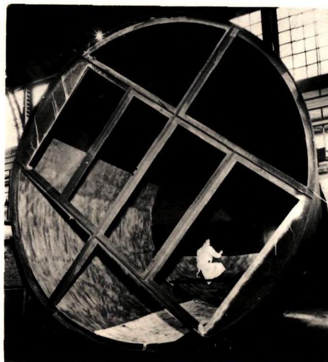
Rolling down natural rubber panels in the interior of a large tank, at the Gaythorn factory.
