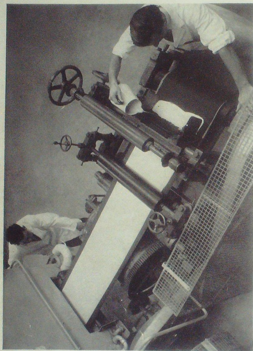
Applying latex foam compound to carpet back. (Courtesy—Revertex [ Frontispiece ] Ltd.)
