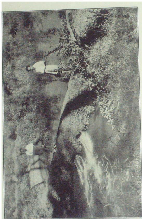
FIG. 3. Hand-operated Sluices made with oil drums in South India.
