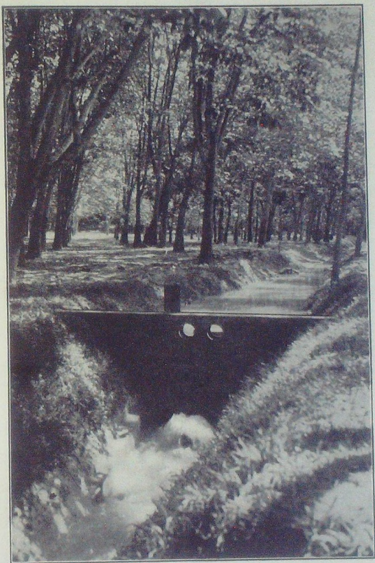
FIG. 1. A de Villiers' Syphon on an estate drain in Malaya.
