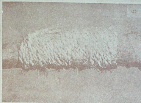
Binding of replaced flap with coir rope.
